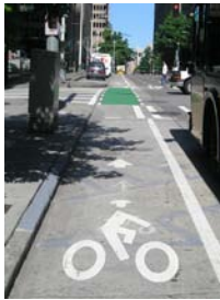
Bike boxes at signalized intersections
