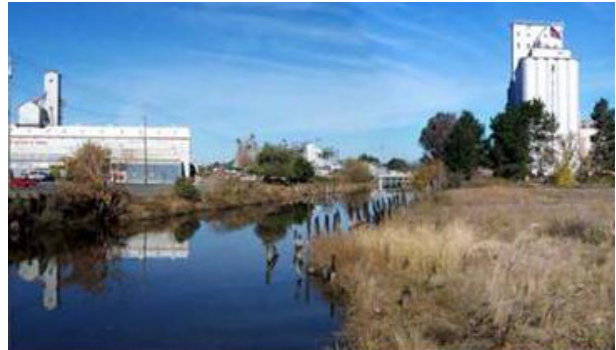
Existing Conditions - Looking north from bridge on E Washington
